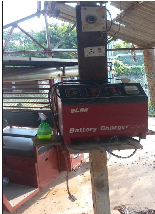
Fig. 4: Charging station for electric vehicles
