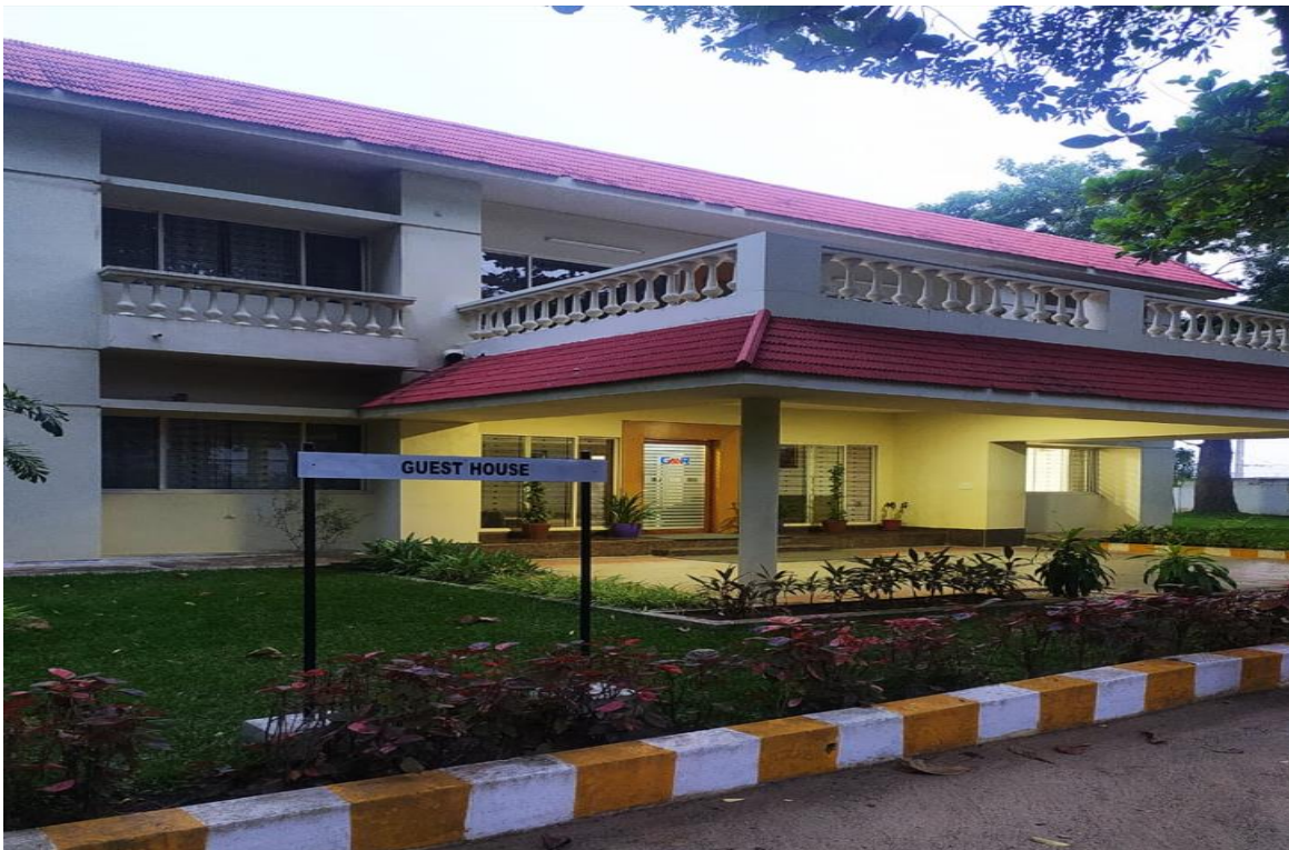
Fig. 1: Guest House in GMRIT campus
