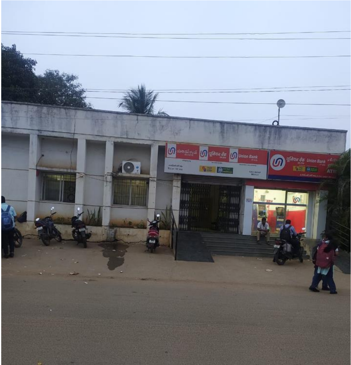
Fig. 2: Bank in GMRIT building
