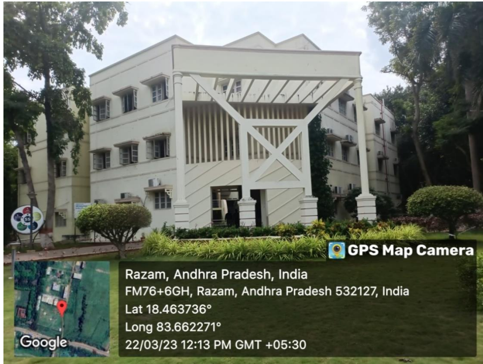
Department of IT and Administration block
